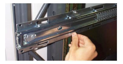
e. Place the server onto the slide mount assembly.
